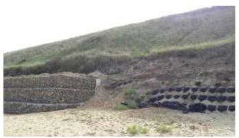
Plate 2.3 Rock-filled gabions installed as emergency protection for the Shell frontage along the BGT frontage (photograph taken on 20/09/2017)
