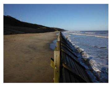
Figure 16-2 Timber Revetment in the study area
