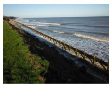
Figure 16-1 Timber Revetment along the frontage in the study area
