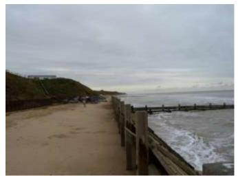
Plate 2.1. The typical timber revetment and groyne arrangement (picture taken on 03/11/2014)
